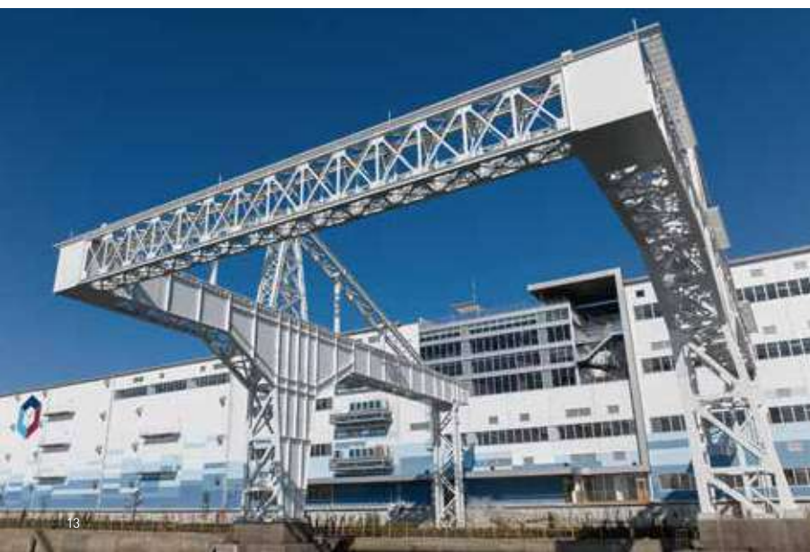
Gantry Crane YOKOHAMA SACHIURA 2
